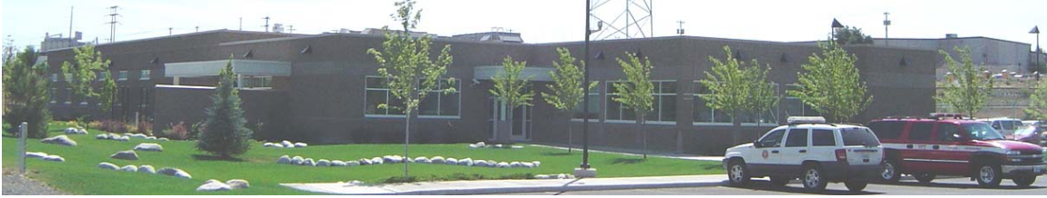
Combined Communications Building (CCB). This building houses 911, the Spokane Crime Reporting Center, and separate dispatch services for Police, Sheriff, and Fire.
